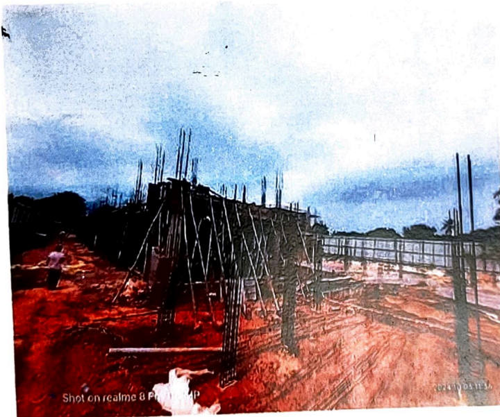
Plate 5: Ongoing construction of hotel
