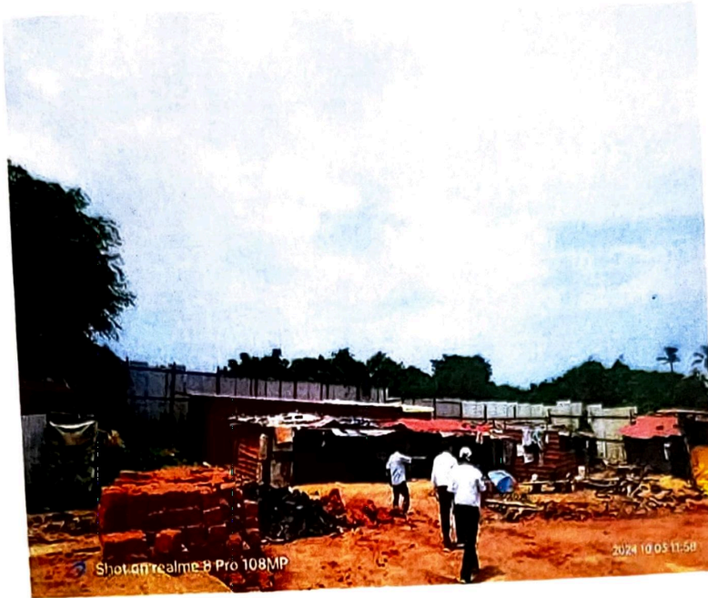
Plate 6: Fencing on the western side of the project site
